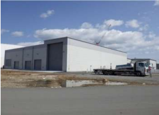
Volume reduction facility
