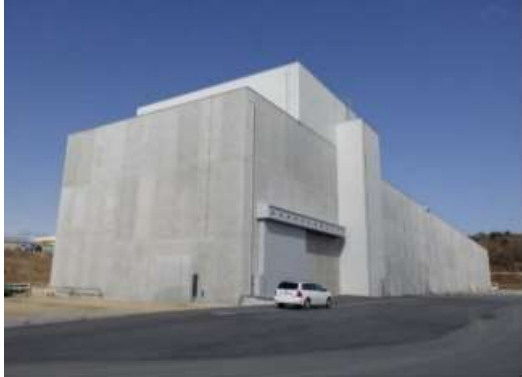
Large waste storage warehouse
